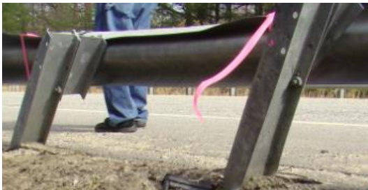
Field Example of Rail Crush
