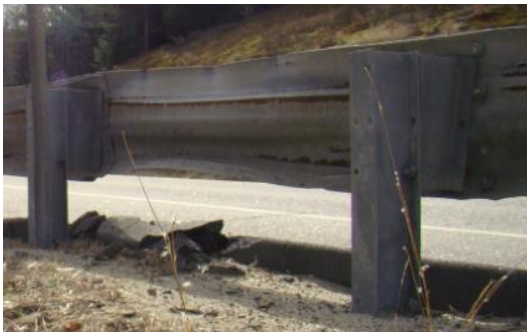
Field Example of Rail Flattening
