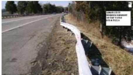
*Rail is bent/pushed more than 18 inches out of line, and/or became less than 24 inches high, or three or more posts are broken/bent over and separated from the rail.\**
