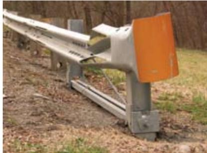
*Post 1 is intact. Rail element is less than 12 inches out of line (non-energy-absorbing end treatment only).*
