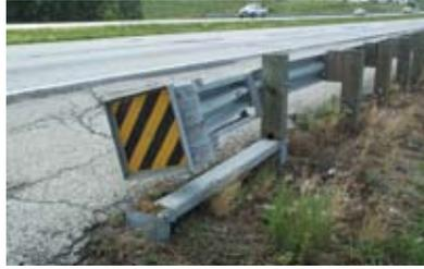
*Post 1 is broken such that full tension is not developed for downstream hits; however, the impact head should absorb most of a vehicle's energy for shallow-angle, end-on impacts.*
