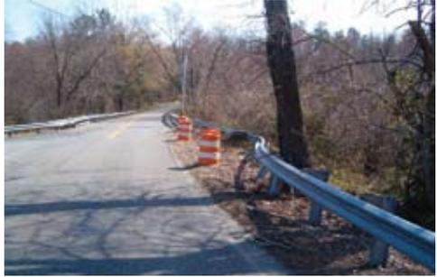
*Drums, as shown, vertical panels, or cones, can be used to warn drivers of the damaged guardrail until it can be repaired.*
