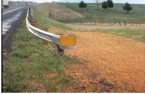
**Modified Eccentric Loader Terminal (MELT)**
