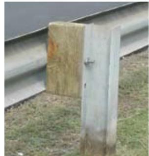
*Strong post W-beam guardrail with wood block and metal post.*
