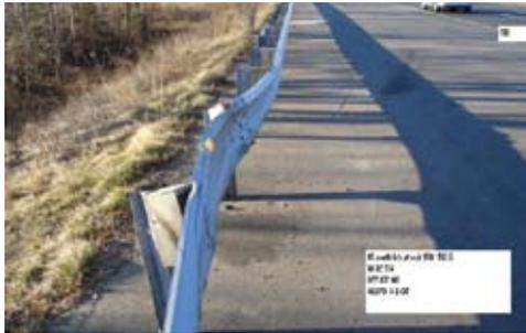
*Rail is bent/pushed out of line less than 6 inches – rail element is intact (no tears and full splices; guardrail height is minimum 26 inches).\**
