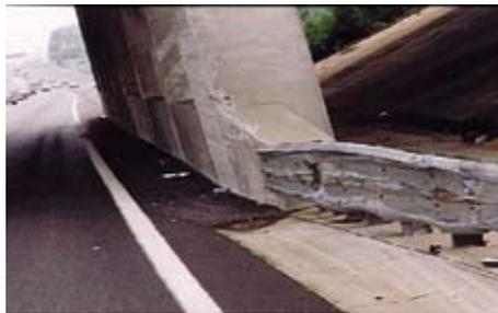
*Rail is flattened and bent / pushed out of line less than 12 inches; rail element is intact and securely attached to the rigid object.*
