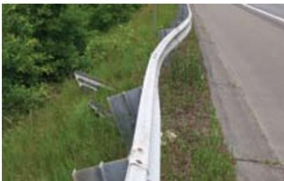
*Rail is bent/pushed out of line less than 12 inches – rail element is intact (no tears and full splices).\**
