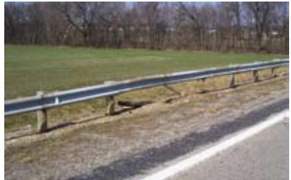
*One or two posts are broken/bent over and separated from the rail – rail element is intact (no tears and full splices).\**
