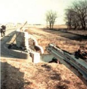
*W-beam element is not attached to rigid object.*
