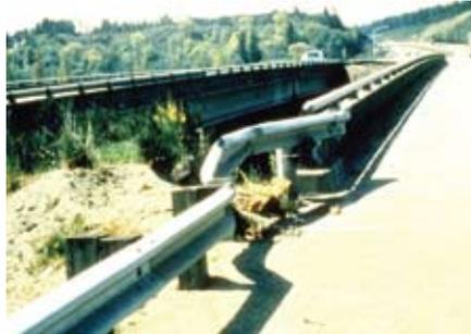
*W-beam is severely pocketed in advance of the rigid object.*
