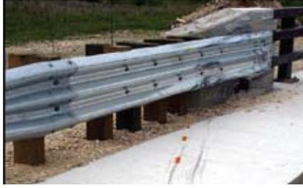
*Rail is flattened / pushed out of line less than 6 inches; rail element is intact and securely attached to the rigid object.*
